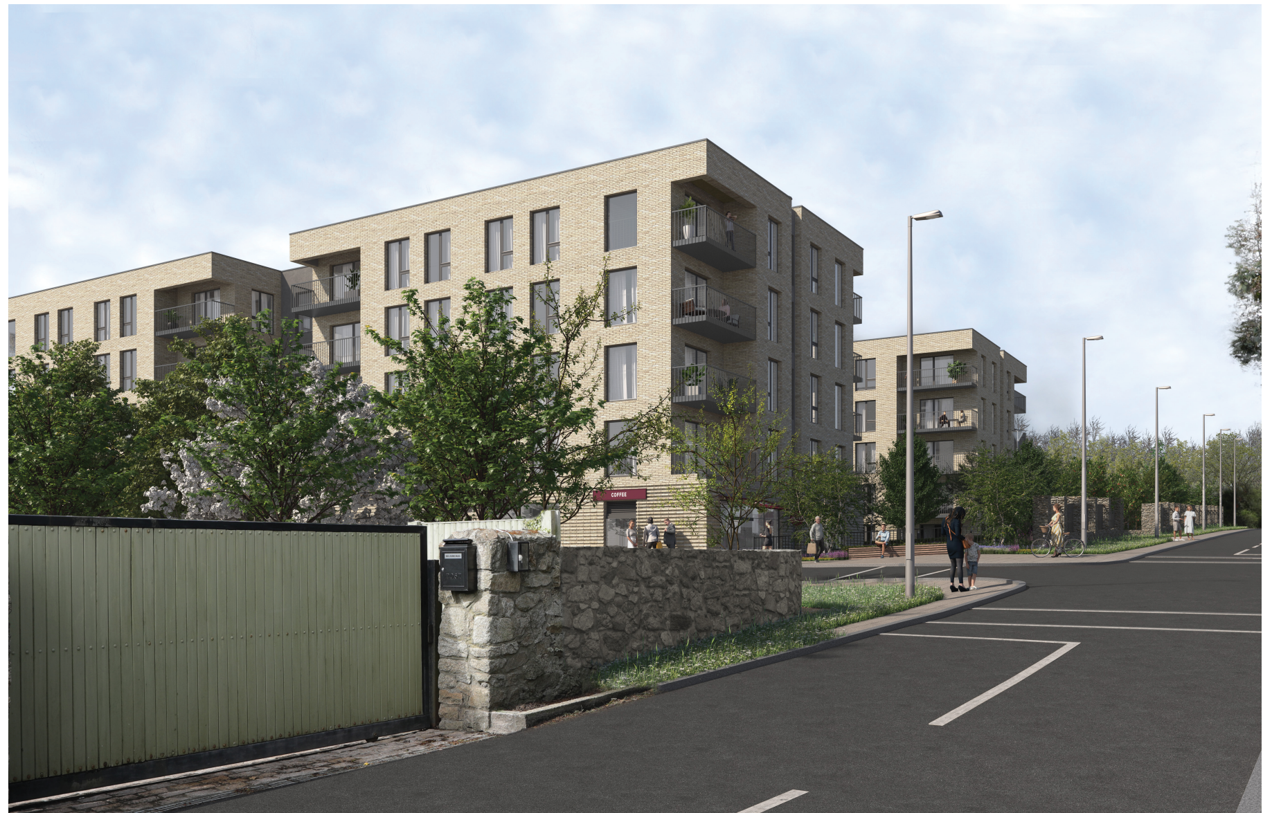
View from Brennanstown Road
