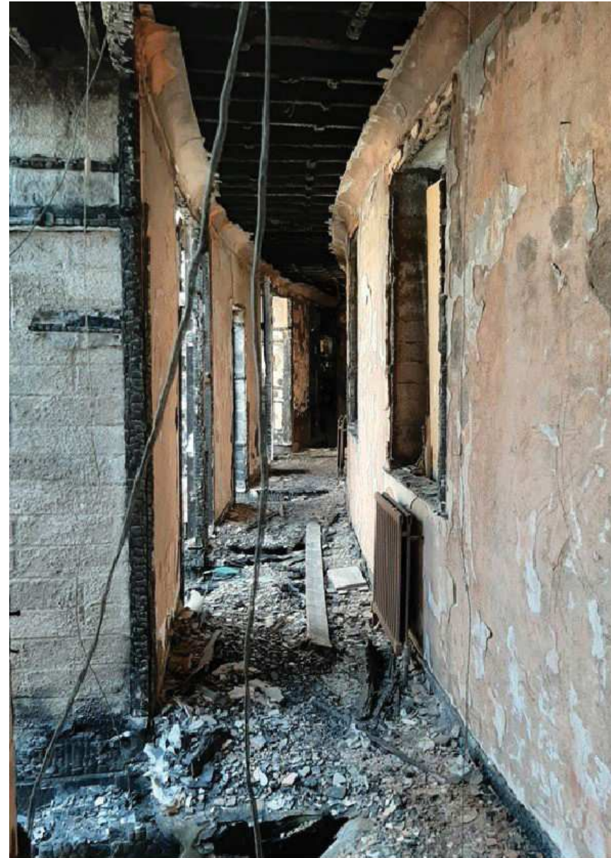
Internal photograph of extension showing current condition - June 2020
