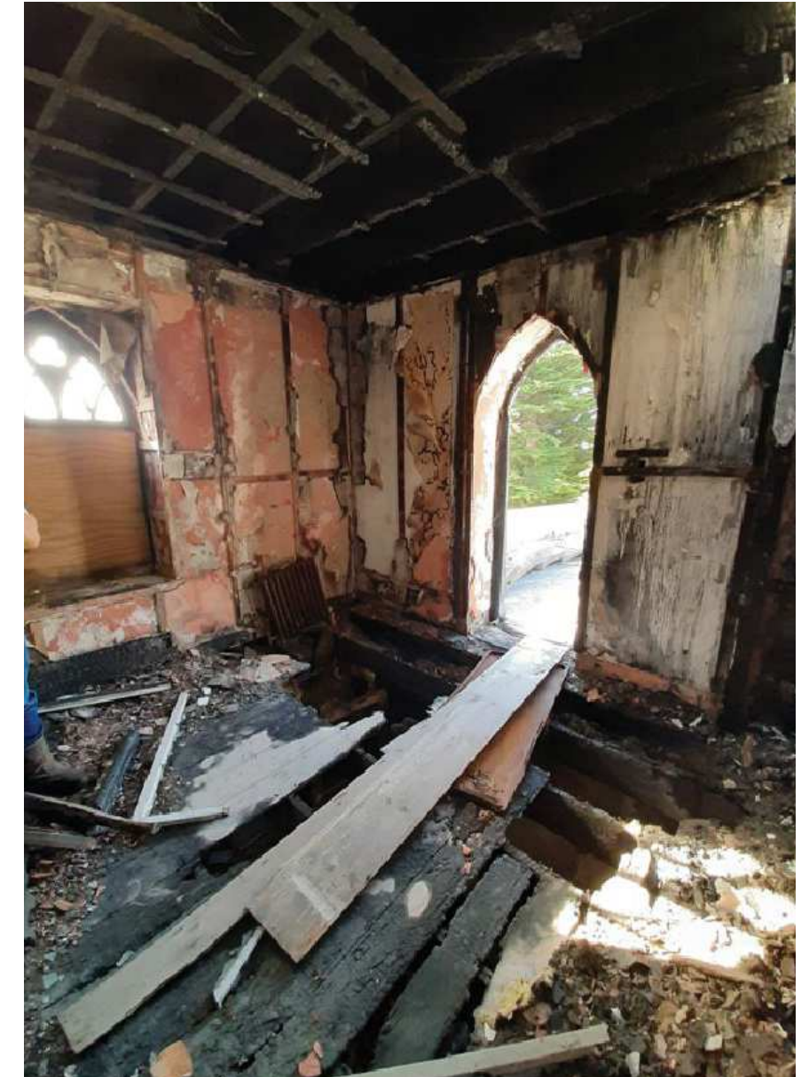
Internal photograph of tower showing current condition - June 2020
