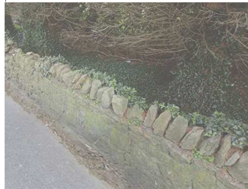
Existing boundary wall.
